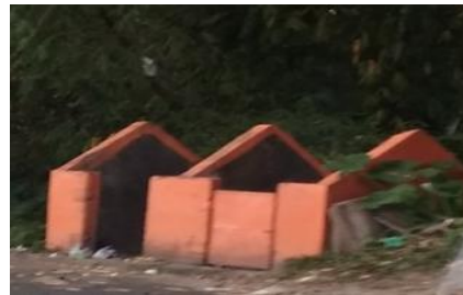
Bak Beton (TSP)
